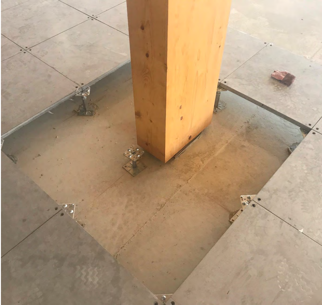
Raised Access Flooring System Installation
